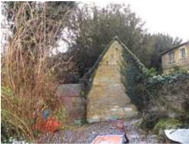
T2 & T3 Toilet block
