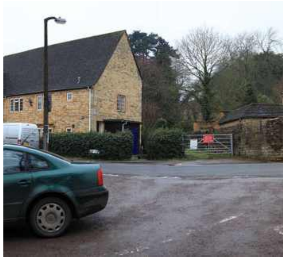
31. View from adjacent to development site to fountain (behind hedge, in grounds of Buchan House). Top of fountain/stone visible but covered in ivy.
