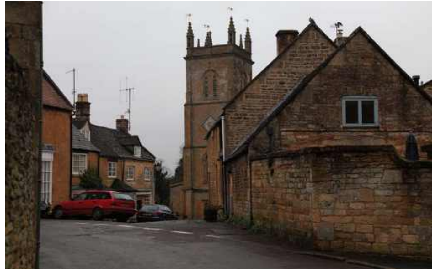
35. View of church tower and The Square - buildings frame the view - creates an entry into the churchyard
