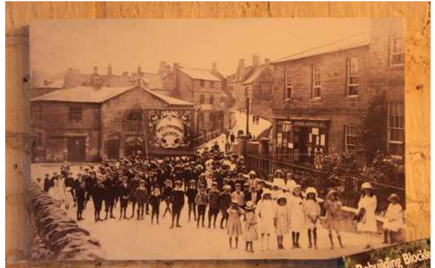
23. Historic photo of shop and former post office. Note 3 storey building to right of shop - now single storey (compare with Image 22).
