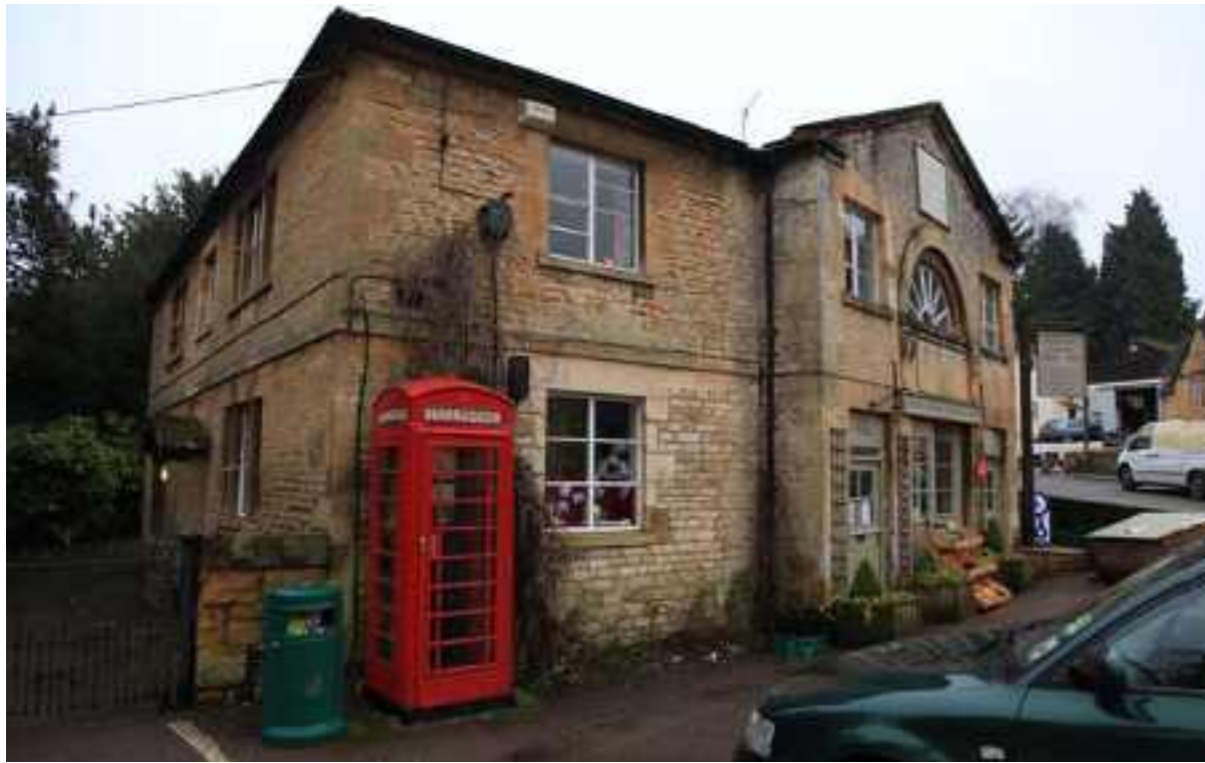
33. View of existing shop, from edge of development site.
