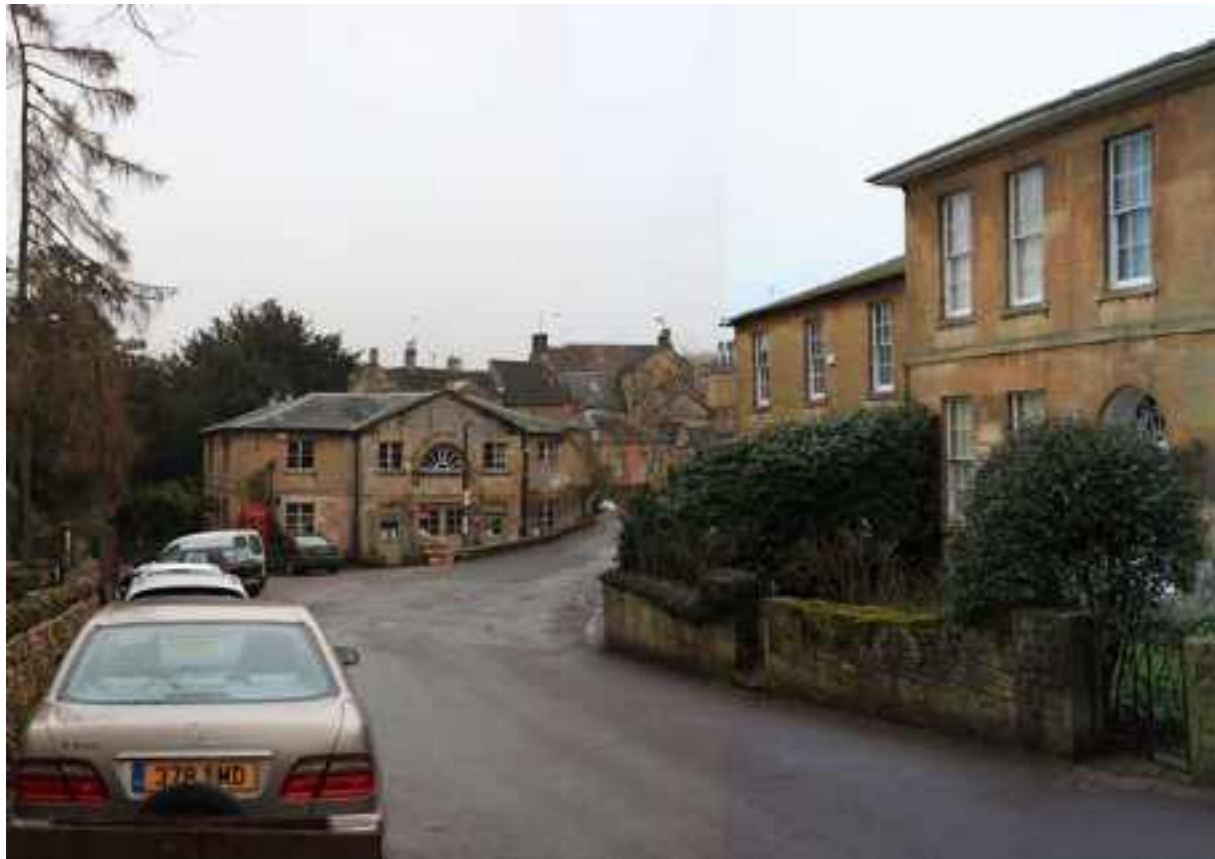
22. View to existing shop; Proposed site to left. Paxton House to right. (Compare view with historic phot, No. 23).
