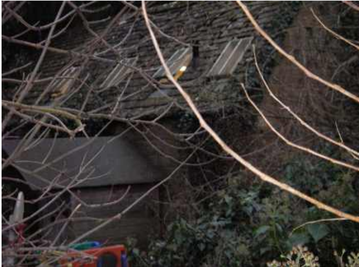
Photo 3 – Rear of existing building
